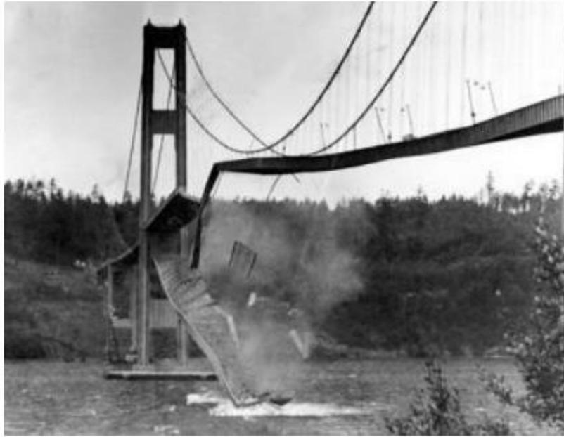
Figura 5 – PONTE TACOMA NARROWS APÓS RUPTURA DEVIDO À RESSONÂNCIA
